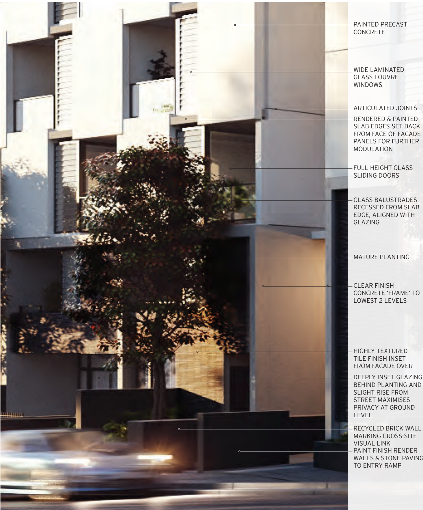
LIVINGSTONE ROAD (WEST ELEVATION) FACADE DETAIL VISUALISATION ILLUSTRATING PROPOSED LAYERING OF FACADE AND ATTENTION TO DETAIL
